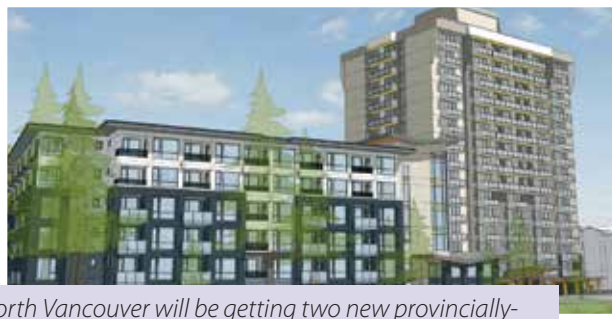
North Vancouver will be getting two new provincially-funded affordable housing projects: a 106-unit seniors' housing complex and a 90-unit family-oriented project.
